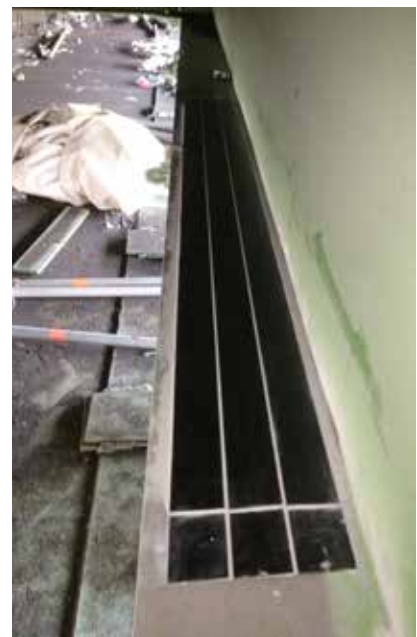
Two layers of Sika CarboDur®
