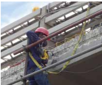
Substrate preparation
