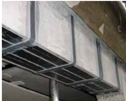
BEAM STRENGTHENING
