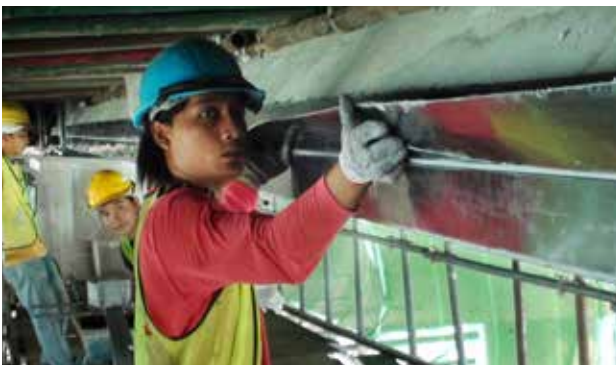
Installation CarboDur®
